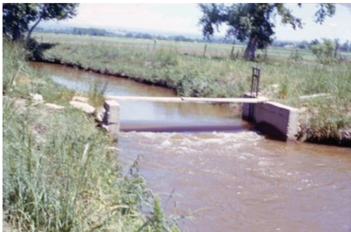
Headgate on Pleasant Valley and Lake Canal, 1941. Photo from the Groundwater Data Collection, Water Resources Archive, CSU.
